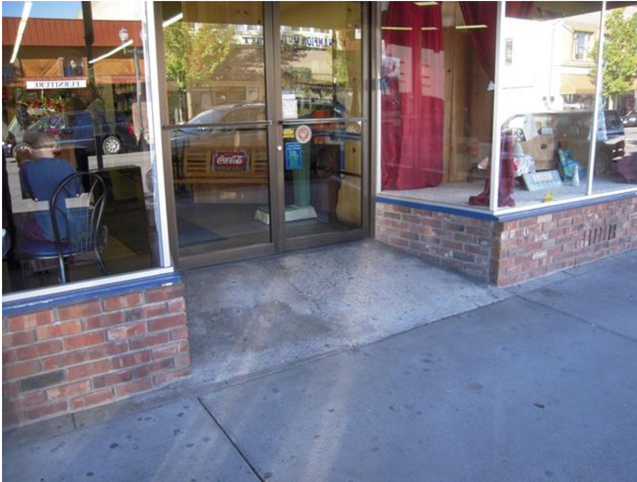
Slope to pharmacy entrance
